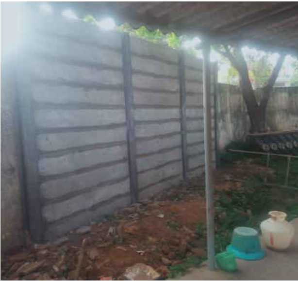
Newly constructed compound wall.
