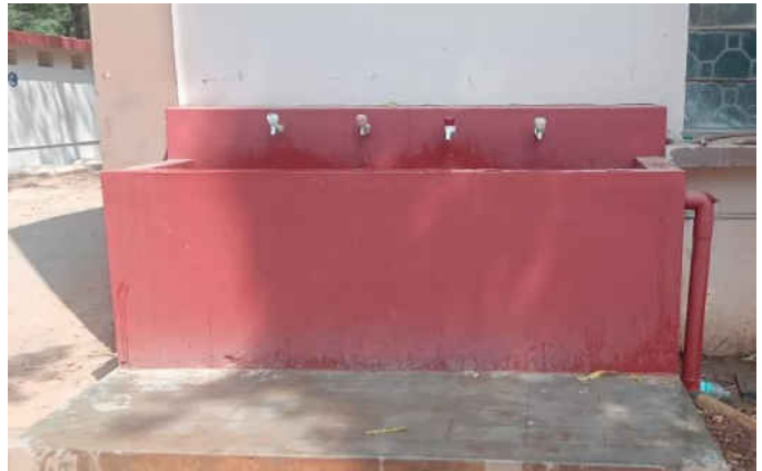
Newly painted water taps area
